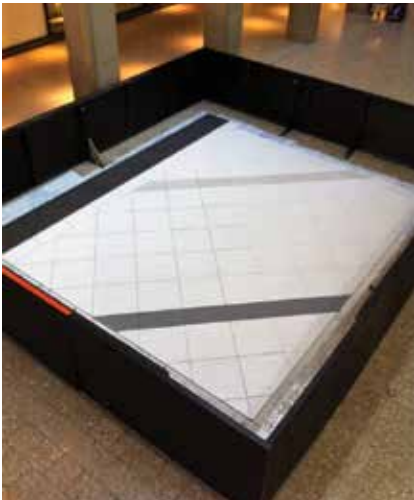
Fig. 3. To manage expectations, the tile supplier or contractor should inform and educate the design professional or end user about variation in the tile, advise them to not select tile from an image, to examine several pieces to understand the range, and to view a dry-laid mockup prior to installation.
